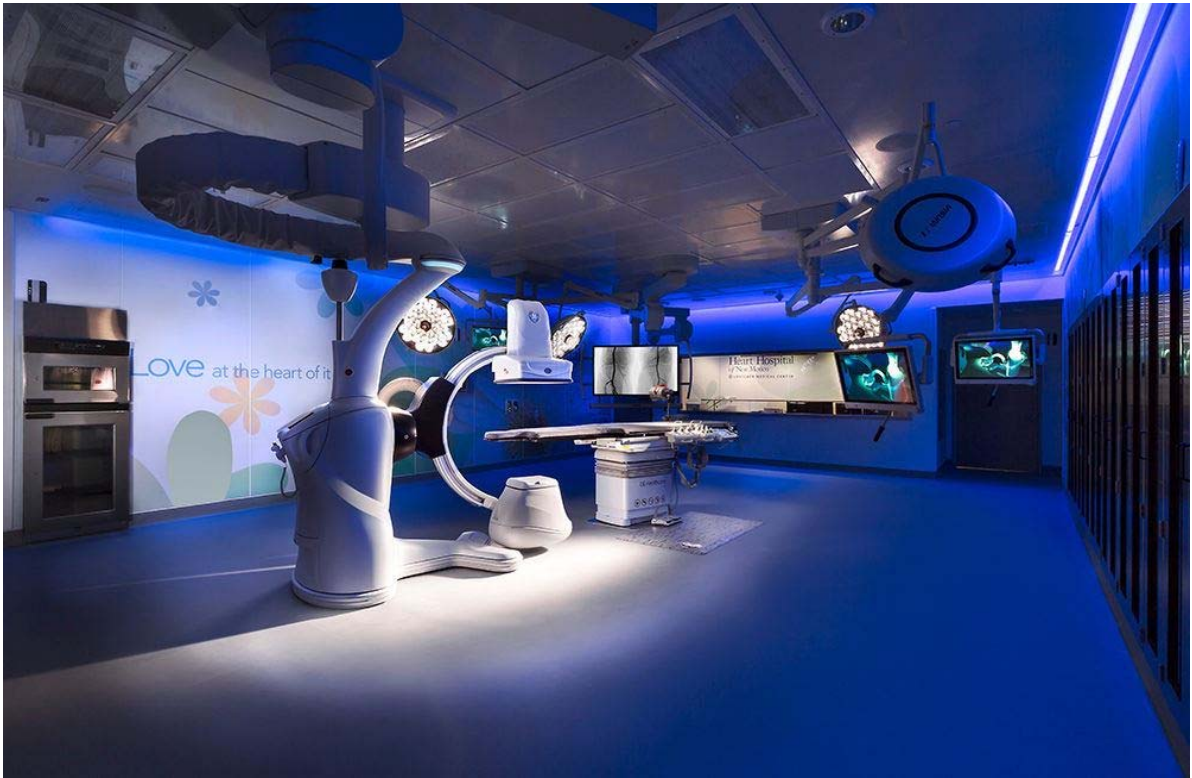
Example of good practices: operating theatre - Heart Hospital of New Mexico, USA
