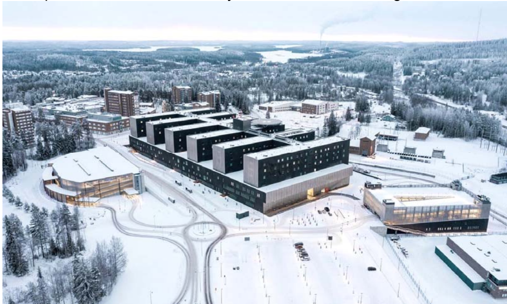
Example of good practices: Hospital Nova, Finland
